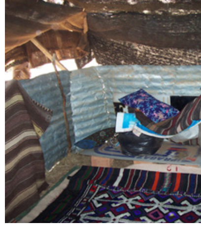
Photos 7-8: Usage of Nylon Sacks and Corrugated Tins Instead of Putte Mats (Photos 7-8: Ayşegül KOYUNCU Archives, İzmir/2008)
